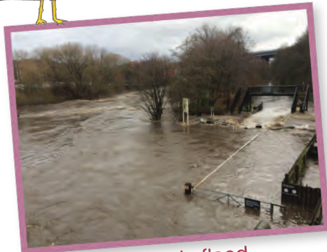
The River Calder in flood
