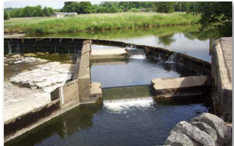
This picture shows the fish pass at low water. Fish can swim up or down these 'steps', which are underwater when the river is flowing fast
