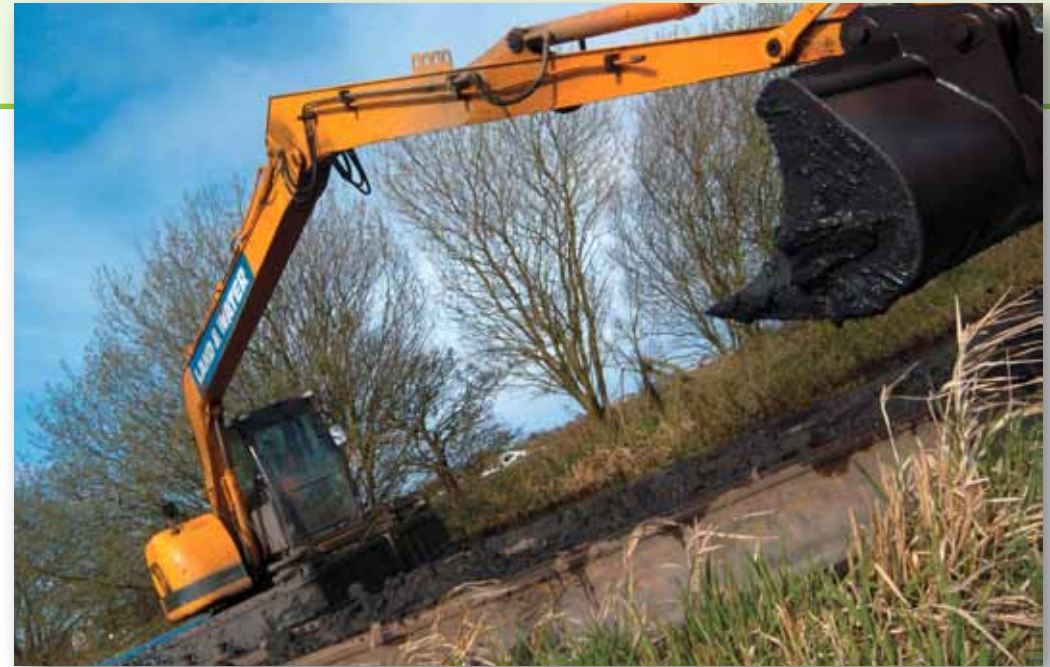
This dredger is removing mud from the bottom of the canal and putting it into a boat, called a mud hopper, to be taken away
