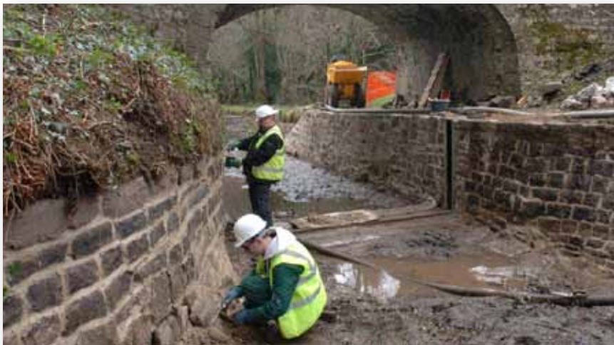
Engineers make sure that stonework matches original materials when doing repairs
