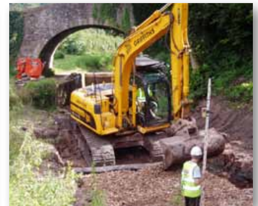
Working on repairs to the Monmouthshire & Brecon Canal
