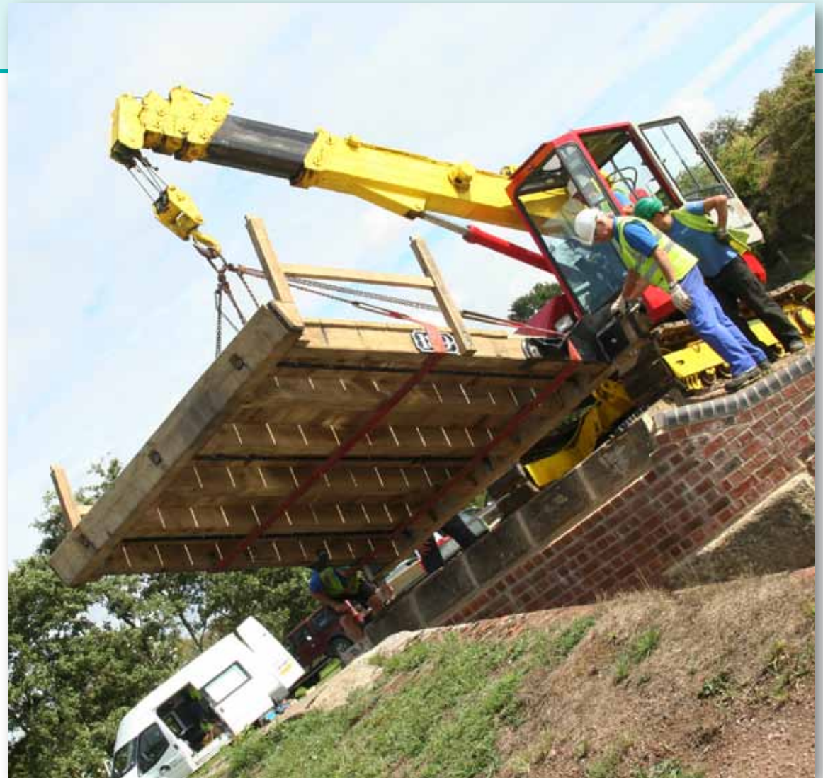
The waterway team is putting in a new lift bridge on the Oxford Canal
