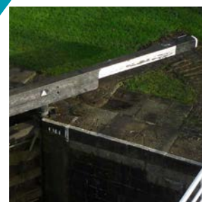
The Lock Gate Balance Beam
